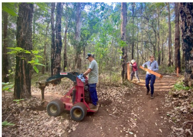
Below: the crew hard at work, installing 42 new jarrah posts throughout the MTB park.
