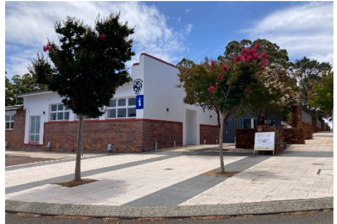
Above: the new Pemberton Visitors Centre will be the meeting point for all social rides.
